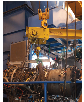
Removal of LM1600™ engine core for essential maintenance
