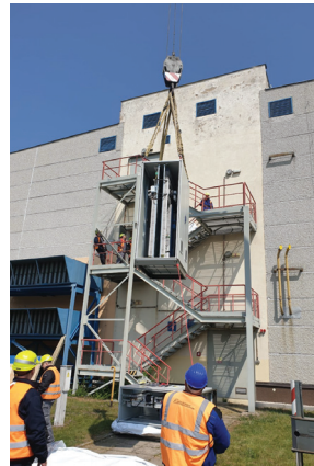
Control panel Crane lift into control room
