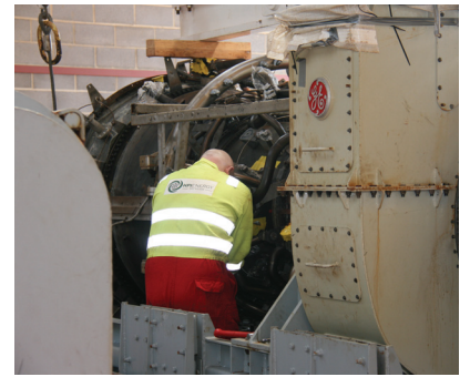
Initial incoming inspection and component removal
